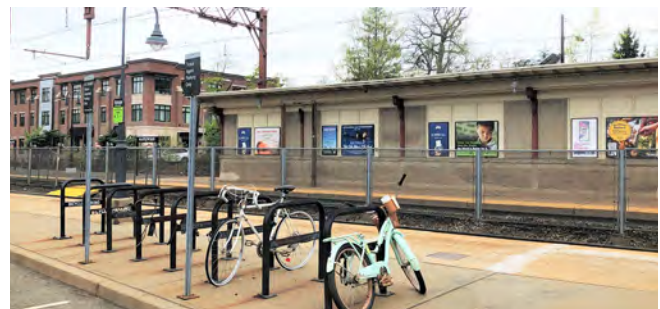
Bicycle Infrastructure at Maplewood Train Station
